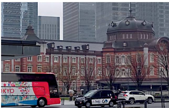
Tokyo Railway Station
